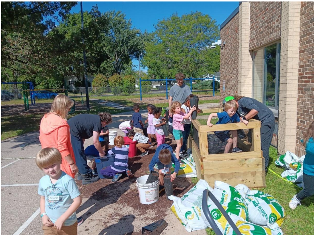
Tree Nursery installation at West Side Elementary in Sun Prairie
